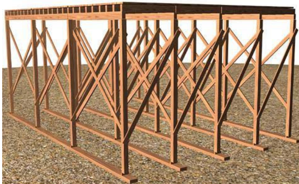
Figure 2: Timber Formwork for Reinforced Concrete Slab
